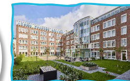
Weissesee nursing home, Germany
