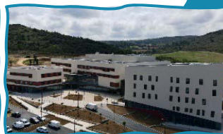
Grand Narbonne Private hospital, Narbonne
