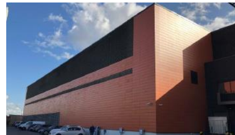
EQUINIX (Portes de Paris Business Park)
