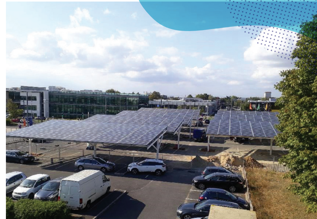
Photovoltaic shade structures, Paris Orly-Rungis business park (Val-de-Marne, Paris Region)
