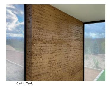
A compressed earth construction method, based on industrial prefabrication, as an alternative to traditional masonry
